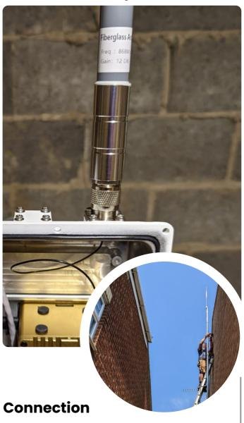
The sma and LMR400 cable easily fit through my air brick and into my loft where my Helium miner resides, antenna installation was very straight forward especially with the light weight and no radials on the antenna to have to deal with.
